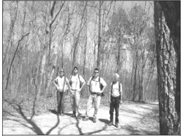
New road connects Peavine Falls Parking Lot to bottom of watershed, just above the falls. Can you say "erosion"? (Photo taken by Laurie Malone 3/21/04)
